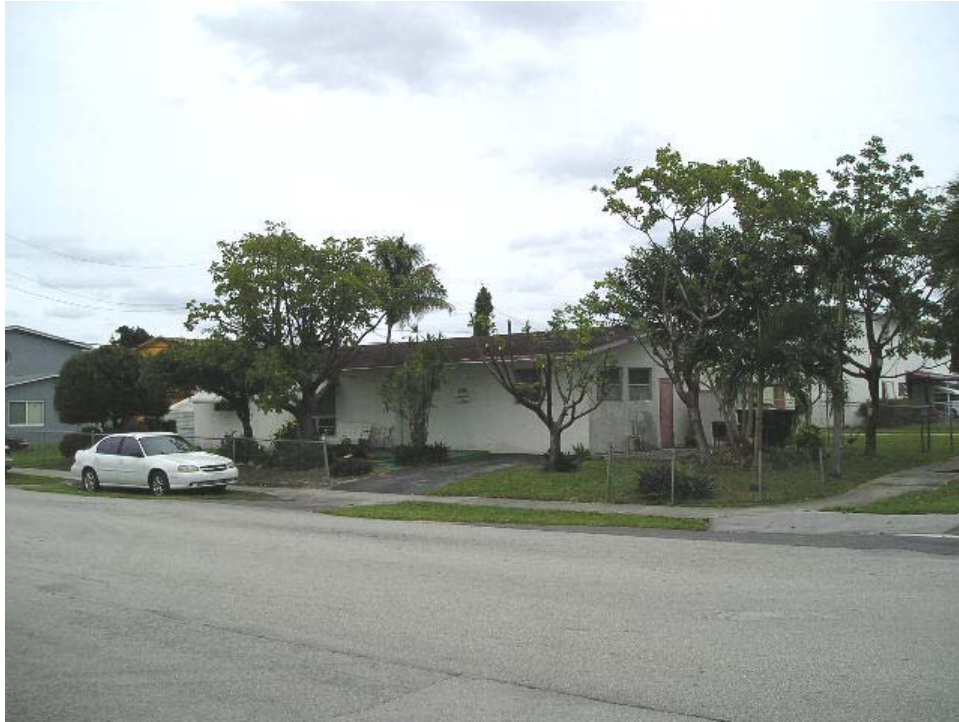
1. VIEW NORTHEASTERLY OF SUBJECT PROPERTY FROM ACROSS SW 12 AVENUE
